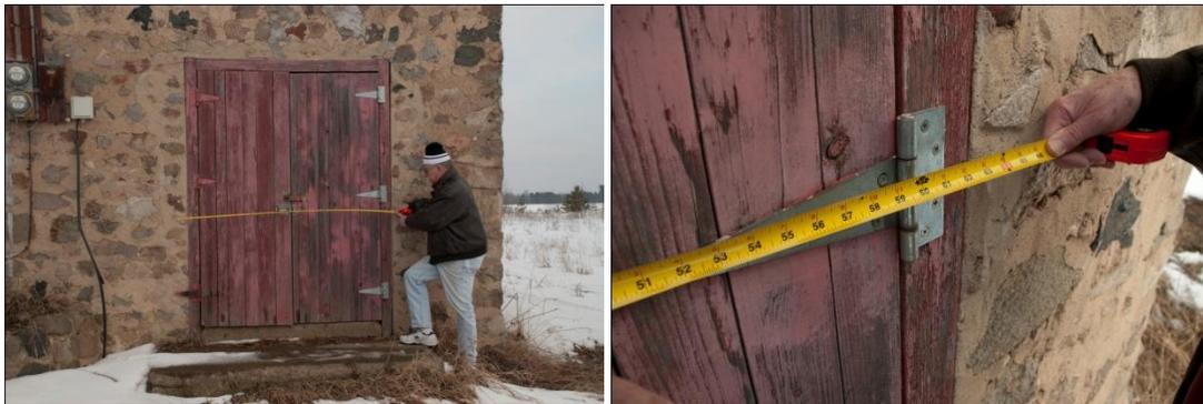
First take a photo of what is being measured (the overall view), then zoom in and get the actual measurement (the specific view).
