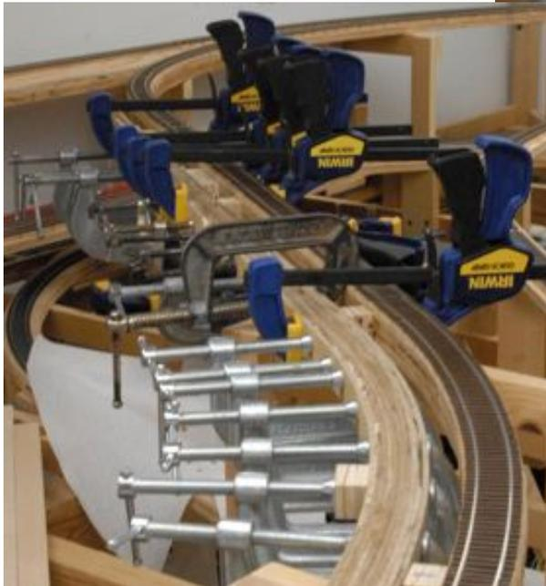
After completing the first of what was to become 11 layers I pre cut the subsequent strips to have the butt joints meet at different support locations. Each spline was added by gluing and clamping it to the previous spline. As I added layers the number of clamps needed grew with the number of layers.
